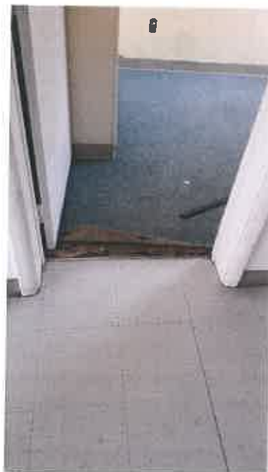
Ab Samples 50,51 Black Mastic under White 12x12 Floor Tile
