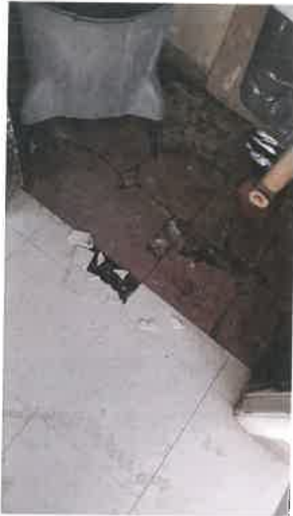
AB Samples 41-46 Red 9x9 Floor Tiles, Black Mastic in Janitor Room
