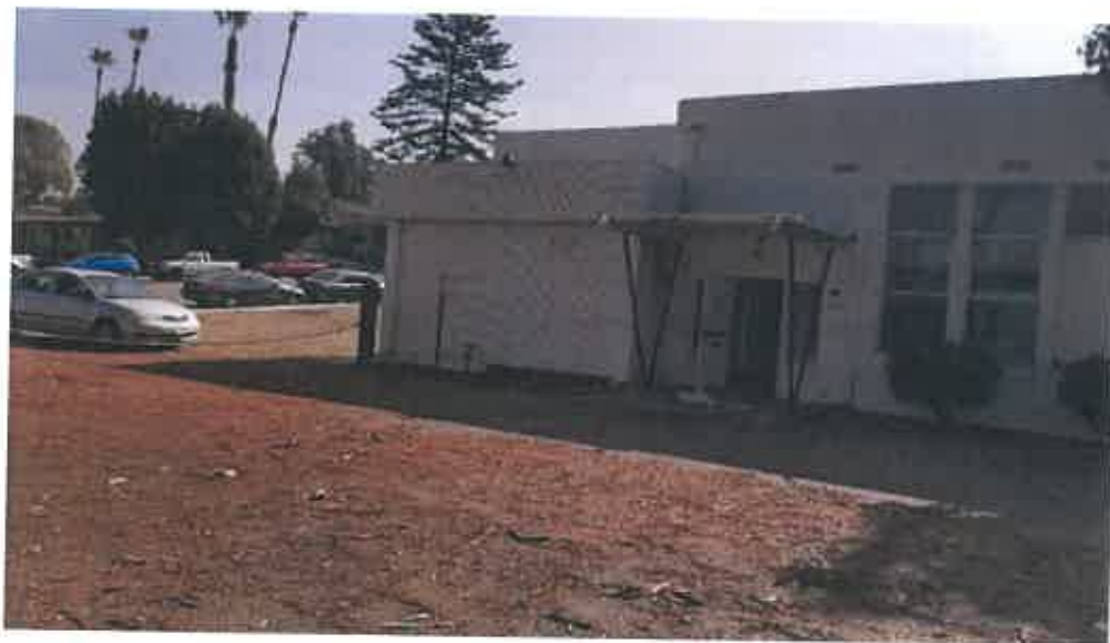
PB- Sample 10 White Lead Base Paint on Exterior Window Frames PB Sample 11 White Lead Containing Paint on Exterior Stucco Walls
