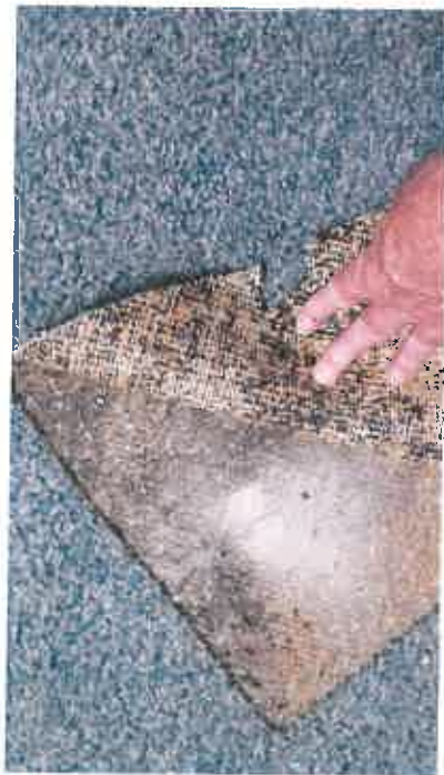
AB Samples 59,60,61 12x12 Floor Tiles, Black Mastic under Gray Carpet
