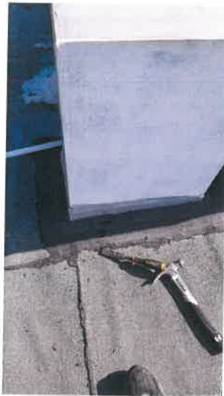
PB Sample 14 White Lead Containing Paint on Exterior Stucco Walls on the Roof
