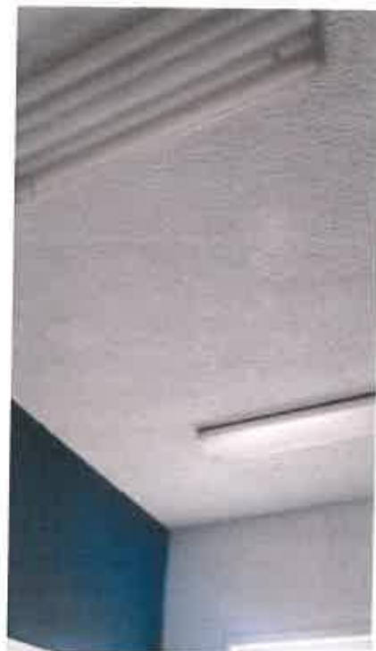
AB Samples 18-20 White Sprayed on Acoustical Ceiling
