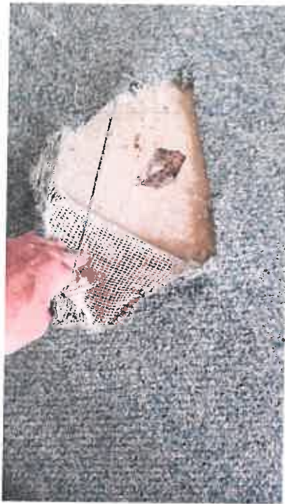
AB Samples 53,54,58 12x12 Floor Tiles, Black Mastic under Blue Carpet
