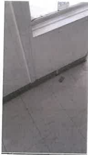
PB- Sample 09 White Lead Containing Paint on Interior Window Frames
